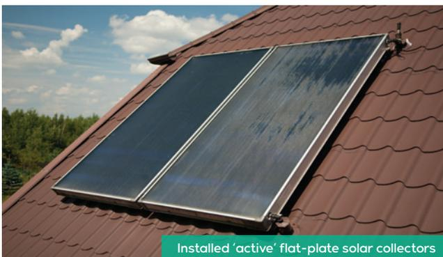
Installed ‘active’ flat-plate solar collectors
